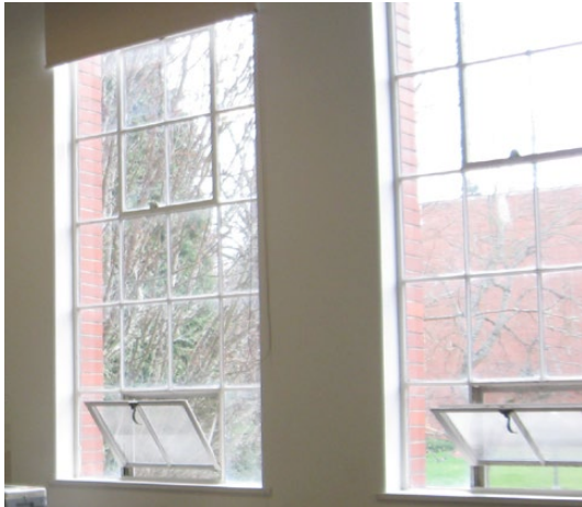
Locking mechanisms on upper operable sections do not match the rest of the windows in Chapman Hall. It appears that they are missing handles.
