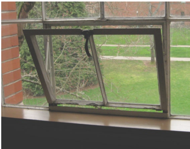
Cracked paint, chipping glazing putty, and rust on southern window in Room 303.
