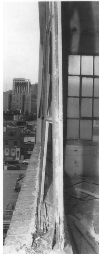
Figure 8. Bowed and corroded window during construction. Photo: Clio Group.
