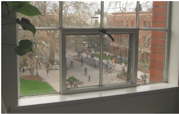
Typical interior condition of west windows.
