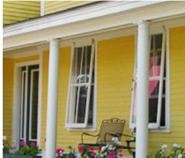
Operable exterior storm windows. Photo courtesy of NPS.
