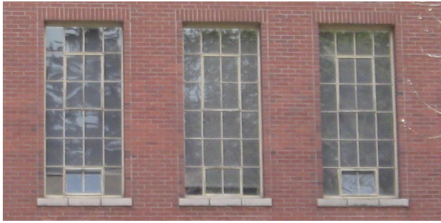
Typical exterior condition of northern windows.
