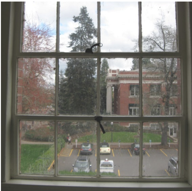
Typical interior condition of eastern windows.
