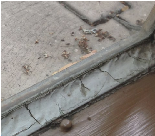
Paint failure found on a window in Chapman Hall.
