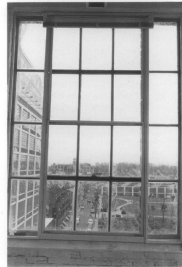
Figure 12. Installed interior triple-track storm window with fixed sidelights. Photo: Clio Group.
