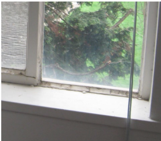
Corrosion found permeating through cracks in the paint and glazing compound on a window in Chapman Hall.
