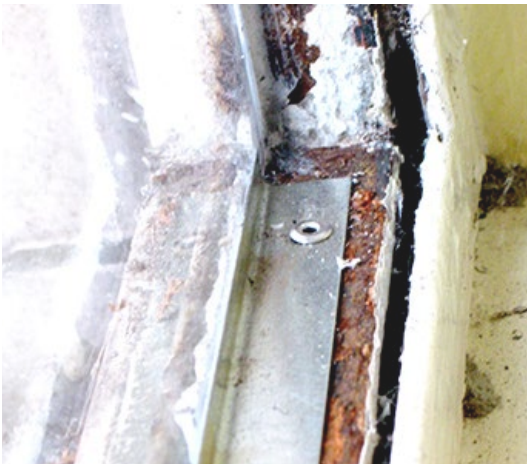
Condon Hall metal section deterioration (none found in Chapman Hall at this time).
