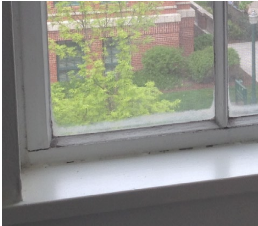
Slight condensation found on interior of window in Chapman Hall. Notice corrosion appearing at joints of steel frame.
