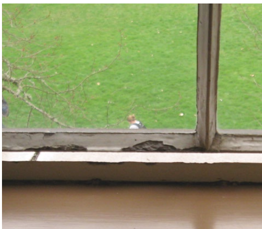
Glazing compound failure found in Chapman Hall.
