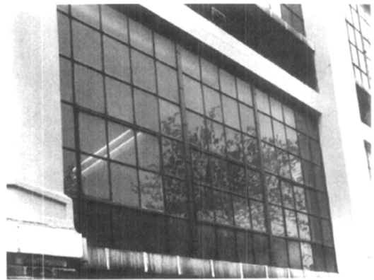
Fig. 10 b. Close-up view of the new replacement steel windows which matched the multi-lighted originals exactly. Photo: Charles
