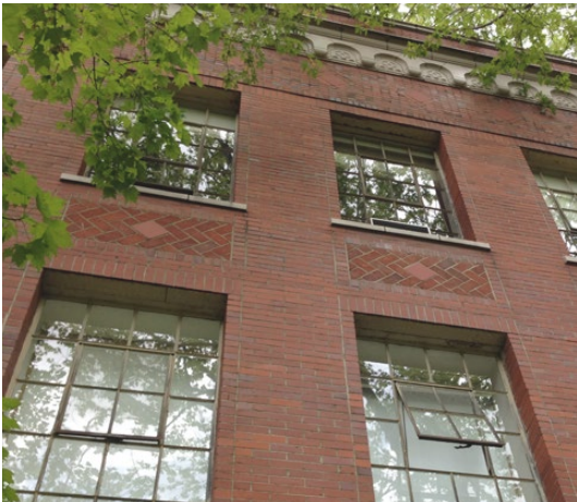
Corrosion of steel lintel in masonry surrounds on Chapman Hall.
