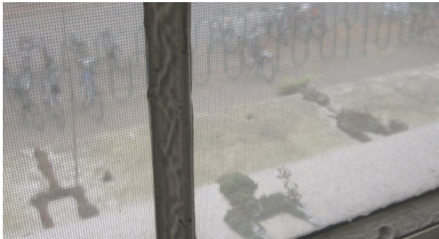
Vegetative growth on northern window sill and typical paint bubbling on interior of northern windows.
