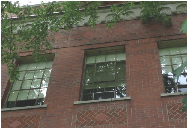
Rust and animal nest on exterior steel lintels of Room 303 windows.
