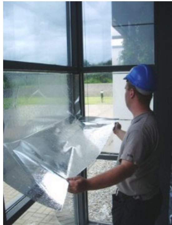
Application of interior surface film. Photo courtesy of Vision Glass Film Products.
