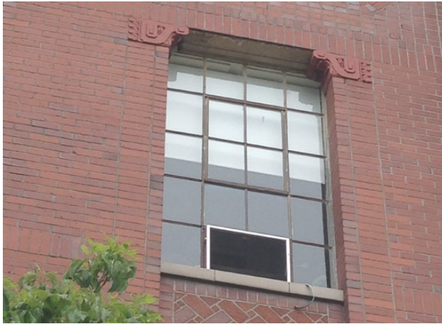
Typical exterior condition of west windows.
