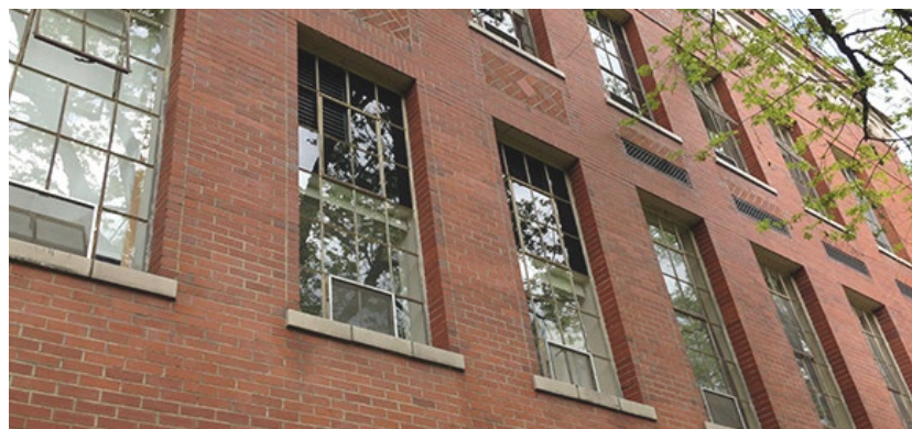
Darkened glazing and vents on south facade of Room 206 as a part of the 2001 Room 207 remodel.
