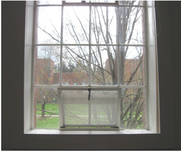
Typical interior condition of southern windows.
