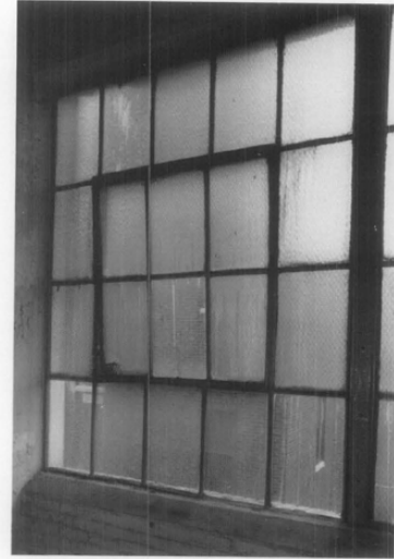
Figure 1. Typical multi-light steel window with ventilator as seen from the interior. This window exhibits typical pre-rehab conditions including sill corrosion, missing hardware and a poorly operating ventilator. Photo: Clio Group.
